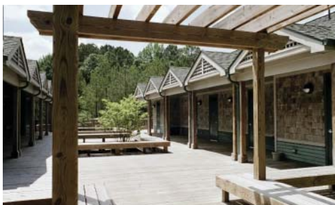
4H Environmental Education Center, NC Construction Admin. for a 226 acre environmental education & conference center comprising some thirteen buildings totaling approximately 35,000 SF
